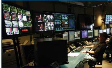
The PBS Network Operations Center (NOC), where network program delivery is managed and monitored 24x7x365
